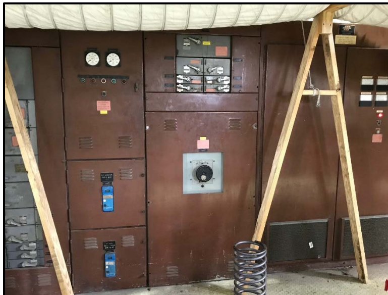
Figure 15 Location of Field Rheostat
